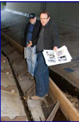
Dr. Alan Webb and Mr. Ross Kapitzke explain how the baffle fishway works through the culvert system in Cubberla Creek
