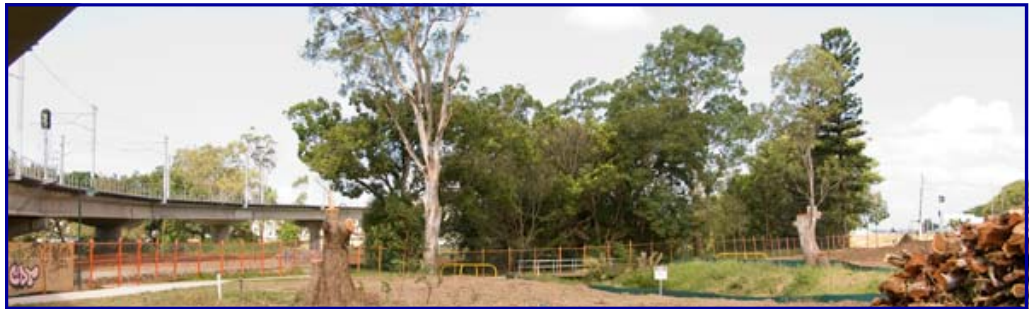
A large area of Kalinga Park being removed to provide room for the Airport-link tunnel portals joining Sandgate Rd and the East West Arterial roadway near Nundah Shopping Centre
