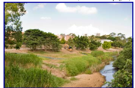
New Greenway replacing the pathways being removed South of the Brook
