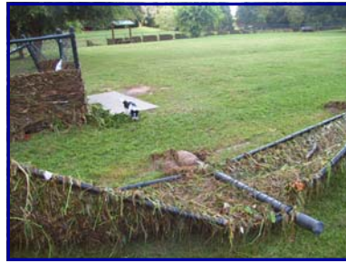
Damage resulting from dam effect of fences at Kalinga Park. (R S-W)
