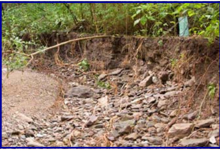
Severe bank damage at Lyn Farrel's place on Cedar Creek
